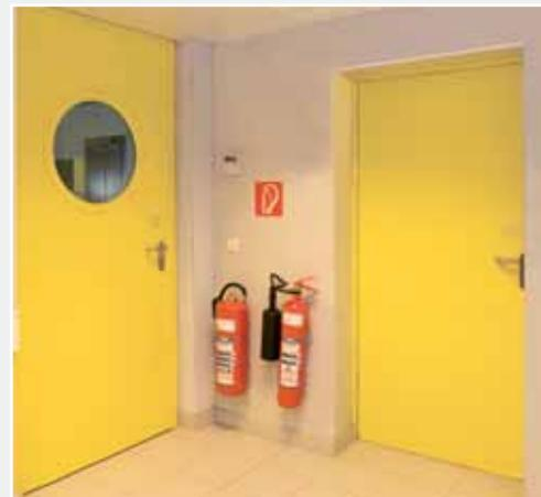
Fire-resistant T30 'Teckentrup OS' doors with a retractable bottom seal guarantee preventive fire and smoke protection.
